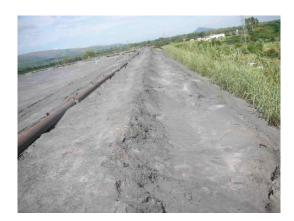
**Result:** The entire tailings complex was treated creating a light crust over the surface, which will prevent the formation of erosion channels caused from heavy rains, allowed for the integrity of the tailings to remain untouched, eliminated the use of an expensive and inefficient sprinkler system and most importantly prevents dust meeting all environmental requirements, improving community relations and providing a safer and healthier work environment.
