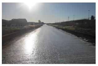
**Result:** a re-constructed surface layer with a newly created wearing course with complete dust elimination, improved skid resistance, total preservation of fines and material, is non-slippery, water and UV resistant, free from the formation of potholes, rutting and corrugation, improved load bearing capacity, increased tensile strength and a reduced environmental impact.
