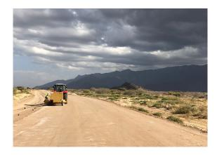
**Application:** The existing surface is ripped, scarified or recycled, then shaped to provide proper drainage, compacted to a smooth finish then sealed with the EBS Soil Stabilizer in multiple coats until the point of refusal is reached. The EBS is allowed to penetrate then the road is opened for traffic
