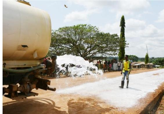
**Application:** The existing surface was scarified, then shaped to provide proper drainage, compacted to a smooth finish then sealed with the EBS Soil Stabilizer using multiple coats until the point of refusal was reached. The EBS was allowed to penetrate then the road was opened for traffic.
