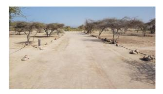
**Project Description:** The areas were constructed by creating a stabilized layer which was compacted then shaped properly to ensure for drainage. The surface was then made smooth and ready for the application of the EBS Surface Seal, which seals and protects the surface from erosion, cracking and any form of deterioration. All work was completed by Soil Solutions and Scan Construction.
