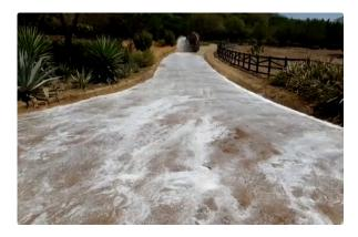
**Application:** The existing surface was skimmed, then shaped to provide proper drainage, compacted to a smooth finish then sealed with the EBS Soil Stabilizer using multiple coats until the point of refusal was reached. The EBS was applied in a manner that allowed for traffic flow during application.
